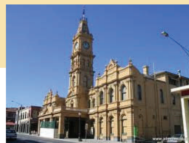
Outside Hawthorn Town Hall.
